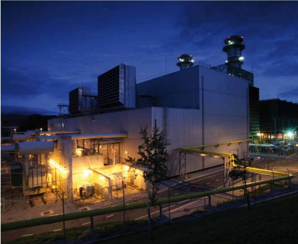
ESB International Power Station at Amorebieta, Spain.
