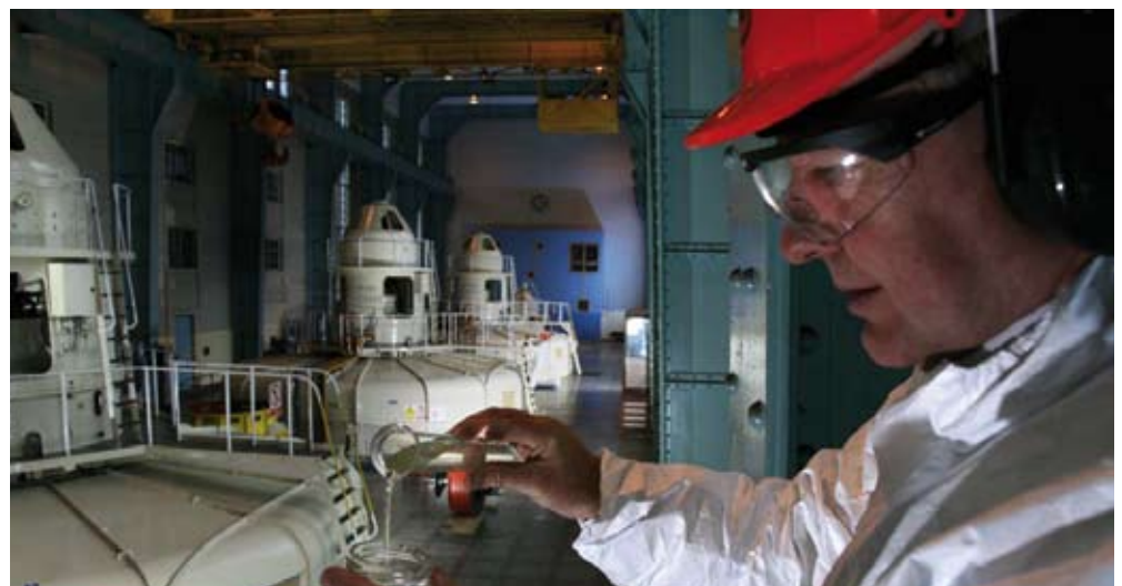
Inside an ESB Powerstation.
