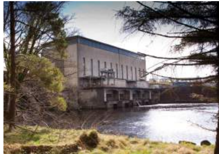
Cliff Generating Station.
