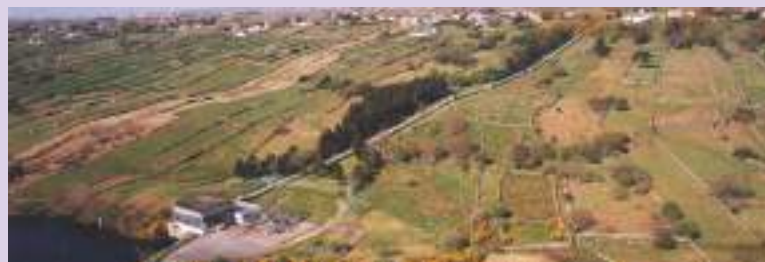
Clady Generating Station, Gweedore, Co. Donegal.
