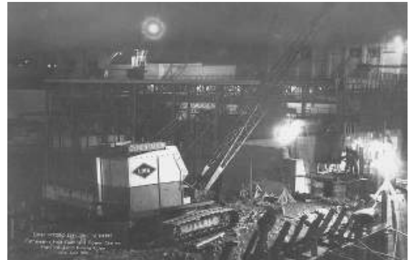
Construction, Cathaleen's Fall at night with crane, 1950.
