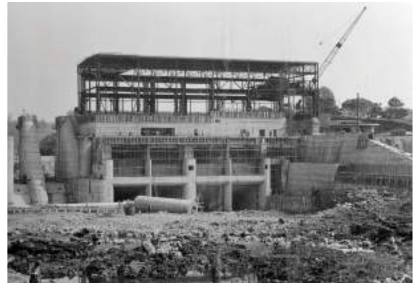
Cliff View, looking upstream to power house mid construction.
